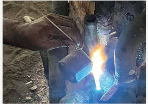
Copper Tube Welding
